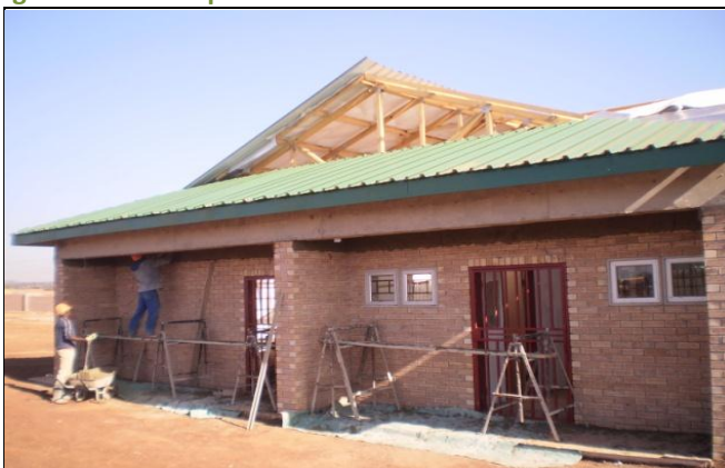
Figure 45: Nellmapius Clinic under construction
