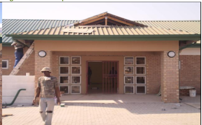
Figure 46: Nellmapius Clinic under construction
